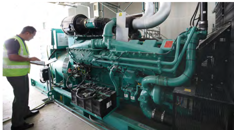
Cummins' legendary KTA50 engine powers the airport gensets.
