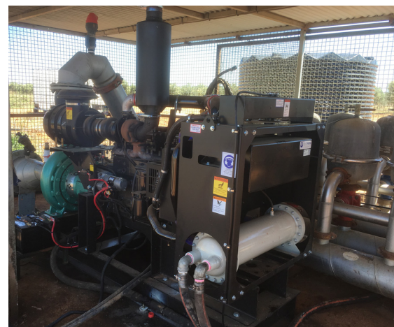
QSL9 engines feature water-to-water heat exchangers instead of traditional radiators.
