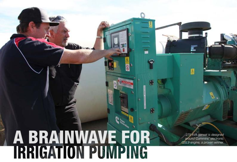
NSW Riverina farmer Ken Brain has achieved more than a 50 percent cost reduction through switching from mains electricity to Cummins diesel generator power for irrigation pumping.
